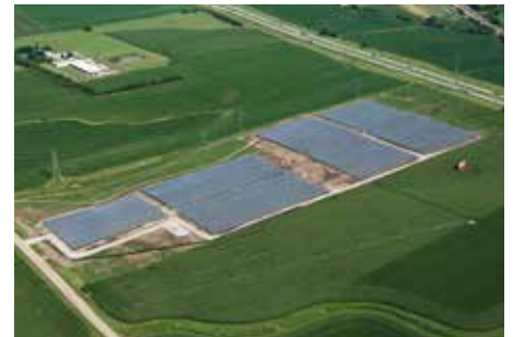
LES' community solar project, located at Northwest 75th & West Holdrege streets, generates 5 MW DC of solar energy.
