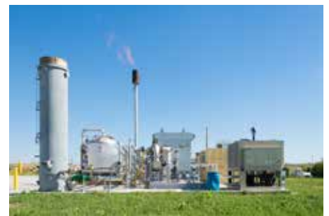
LES' 5-MW landfill gas-powered facility uses methane fuel supplied from the Bluff Road Landfill.
